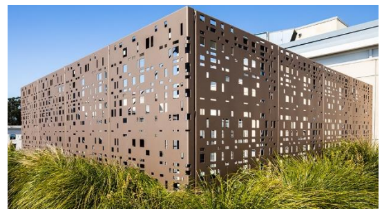
Ground-mounted equipment screening
