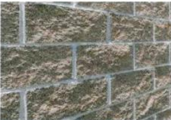
Figure 4 Masonry (Architectural Finish)
