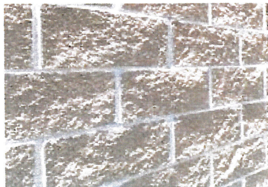
Figure 4 Masonry (Architectural Finish)
